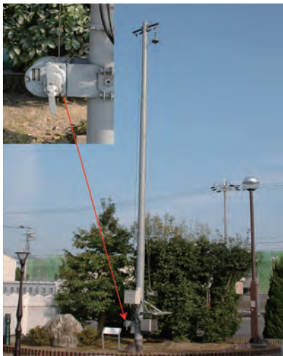
Fire fighting hose hanger
