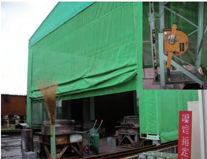
Lifting a blocking sheet at warehouse doorway
